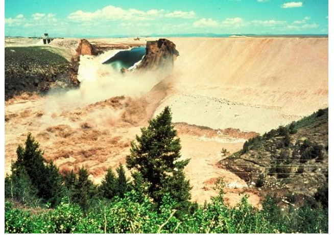
About 4-5 hours later, the water could not be stopped.
