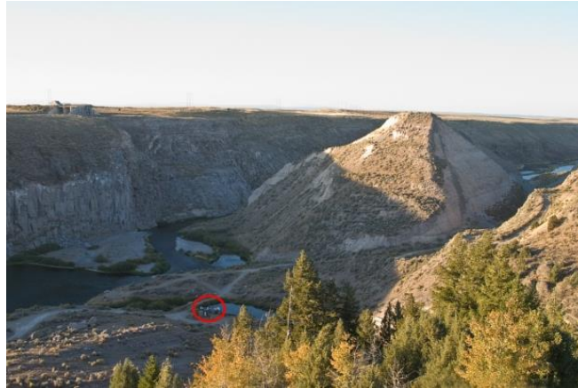
All it takes it one tiny crack in the dam, and the whole thing comes crashing down very quickly.
